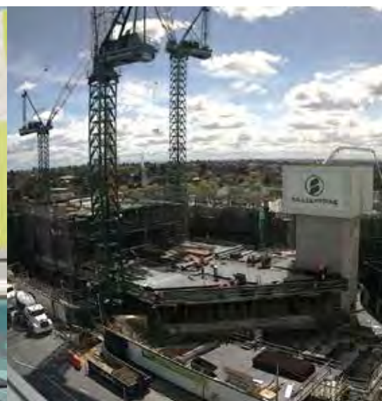
Construction of the Box Hill Hospital
